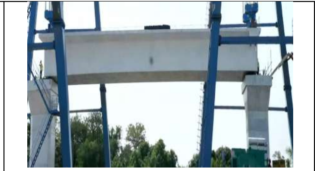
Fig 2: Casting of Full Span Box Girder
