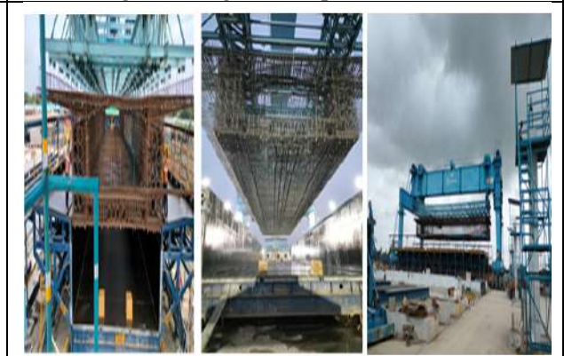
Fig 2: Casting of Full Span Box Girder
